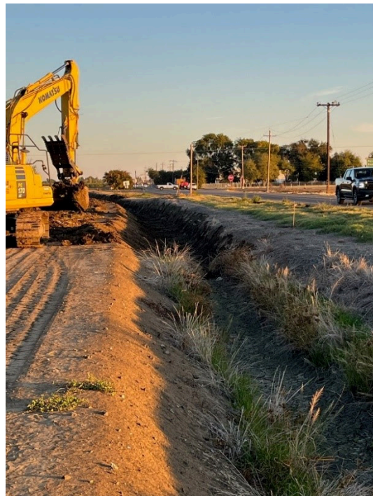
RD2068 Re-shaping Lateral 1 – Fall 2023
