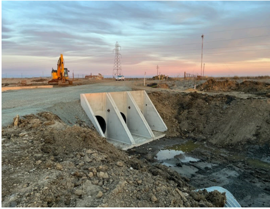
Delhi Road – V-Drain Crossing Replacement – November 2024 A joint effort between RD2068 / Solano County / Dixon RCD
