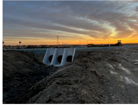
Delhi Road – V-Drain Crossing Replacement – November 2024 A joint effort between RD2068 / Solano County / Dixon RCD
